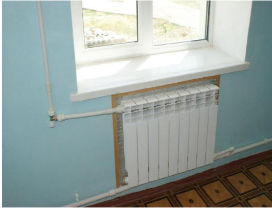
Fragment 7: Installation of aluminum radiators with thermal regulation valves
